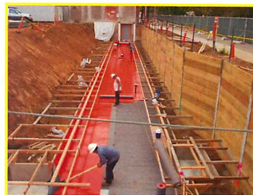
BELOW-GRADE WATERPROOFING INSTALLATION INSPECTION
