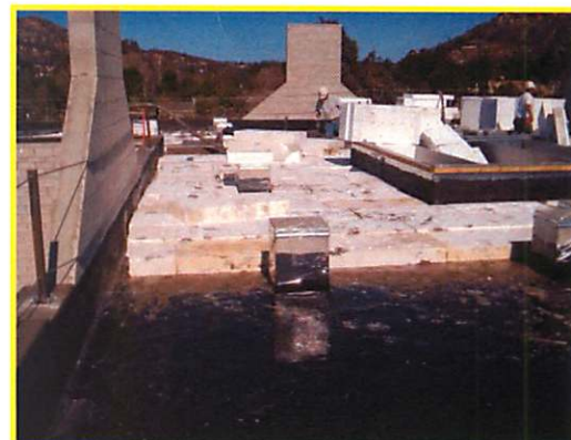
ROOFING FLOOD TEST SCRIPPS HOSPITAL, LA JOLLA
